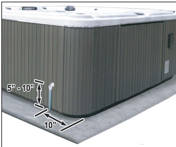
**Method 1:** Feeding the conduit through the cement slab to line up with your spas front right corner.
